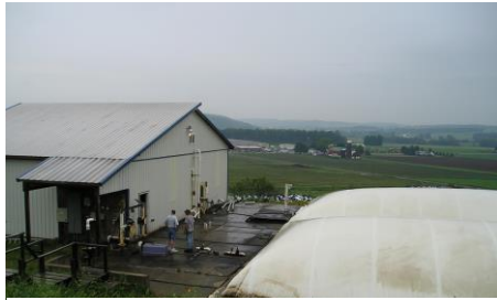
Figure 3. Plug flow digester with flexible cover at a 650-cow dairy in New York.
