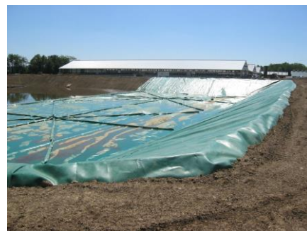
Figure 2. Newly installed flexible cover on ½ lagoon at 700-cow dairy in Ohio.
