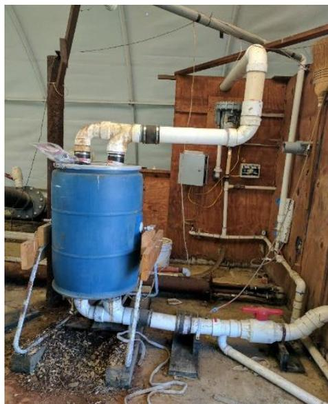
**Figure 1. Iron oxide scrubber**
