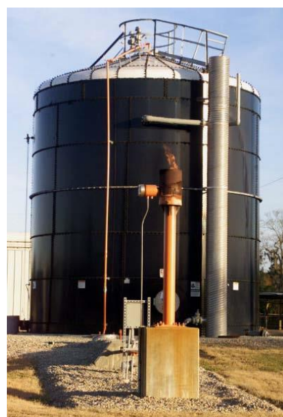
Figure 6. Fixed-film digester operating in Florida. (Photo credit: Ann C. Wilkie)
