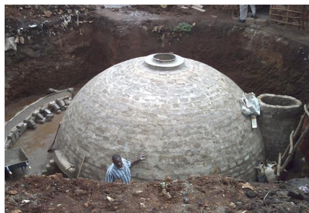
Figure 10. A fixed-dome digester under construction in Africa. (Photo credit: Bustler)
