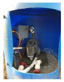
Figure 1. Air Injection Pump
