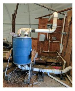
Figure 1. Iron oxide scrubber
