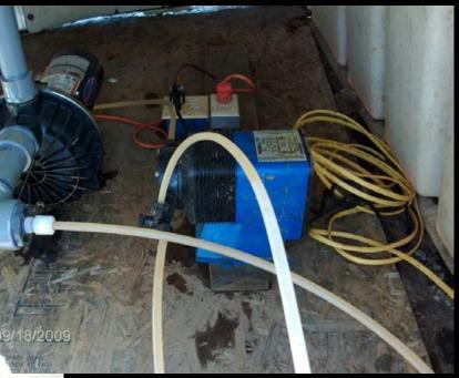
Digester Influent Additive: <u>Ferric Hydroxide - Fe (OH)</u>3
