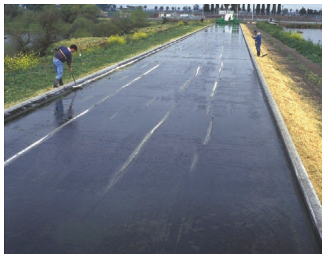
Figure 2. Pilot-scale ATS tertiary wastewater treatment system in Patterson, California. See Craggs and colleagues (1996).
