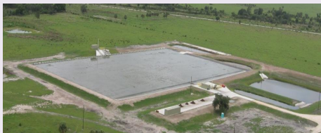
3 acre ATS system in Florida used for phosphorus and nitrogen reduction on a eutrophic stream
