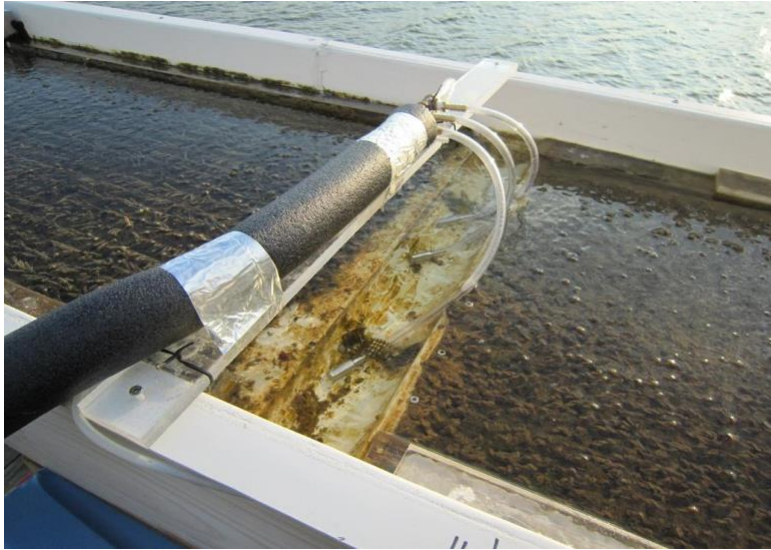
Figure 13: Stainless steel injectors at the 50% injection trough. Note the short tube exiting the neoprene insulator just to the left of the CO 2 tubes; this is the drip point for the nutrient solution. The 75% injection point is the same, although without nutrient injection.
