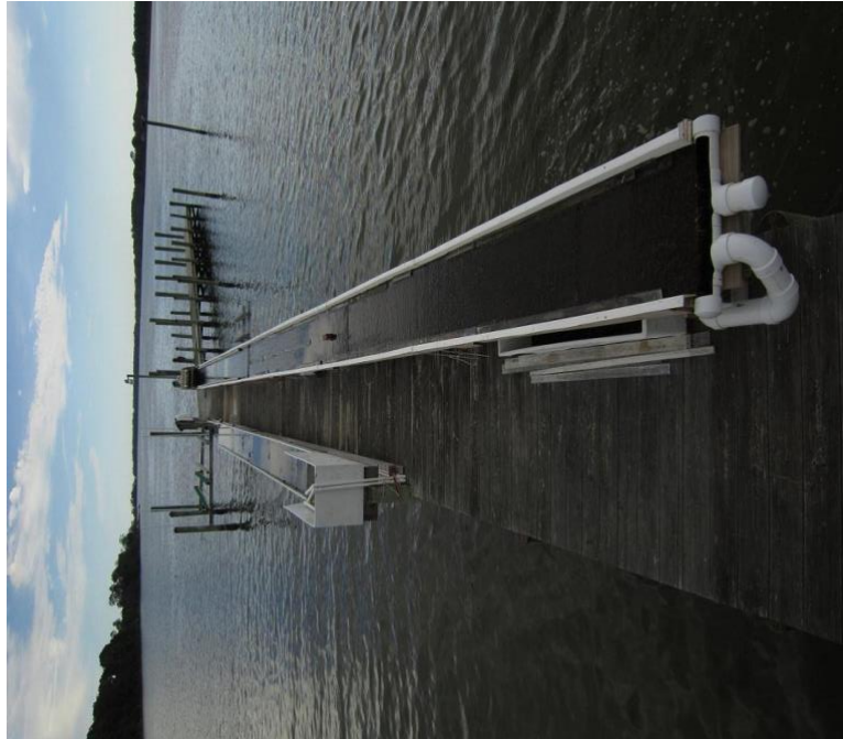
Figure 1: Flowway #1 (left) and Flowway # 2 (right) on the Great Wicomico River in the Central Chesapeake Bay. This is a mesohaline river, with salinities at about 12-15 ppt. Two separate, submersible pumps, established on the outer part of the flowways provide a flow of about 20 gpm to each. The pumps are on separate electrical circuits, with an automatic backup electrical generator. During the term of operation of these two flowways, no interruption of water flow has occurred, except during short term, non-drying harvests and maintenance.
